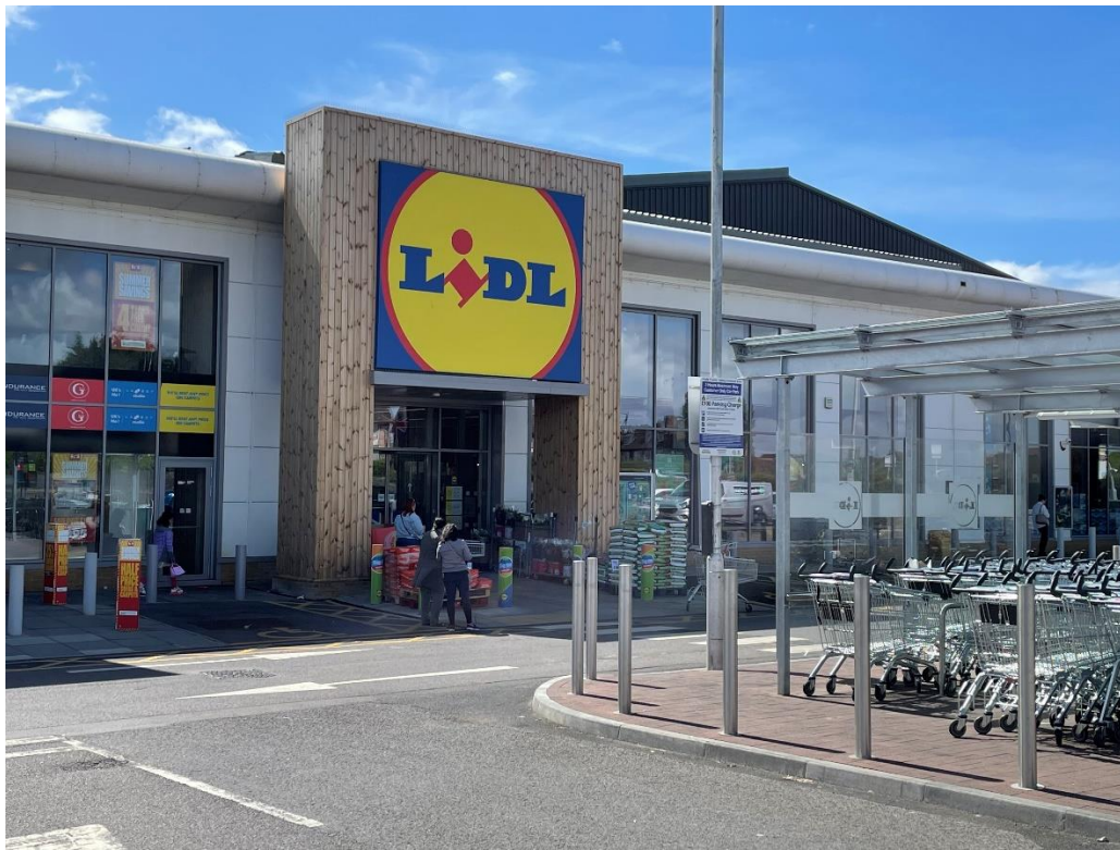
Front door access to the site building.
